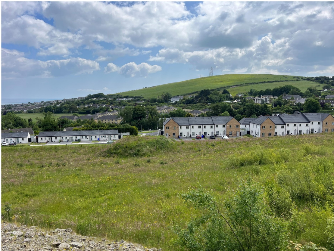
Photo 2. Overview of the site at rear of existing housing in Phase 1.
